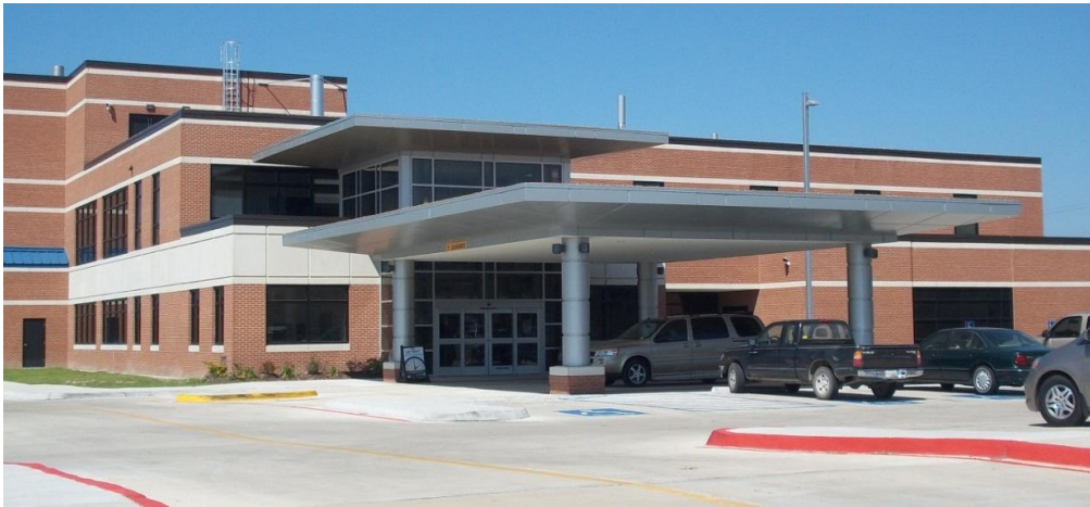
New entrance to West Calcasieu Cameron Hospital – Part of Phase 1 of the expansion plan
